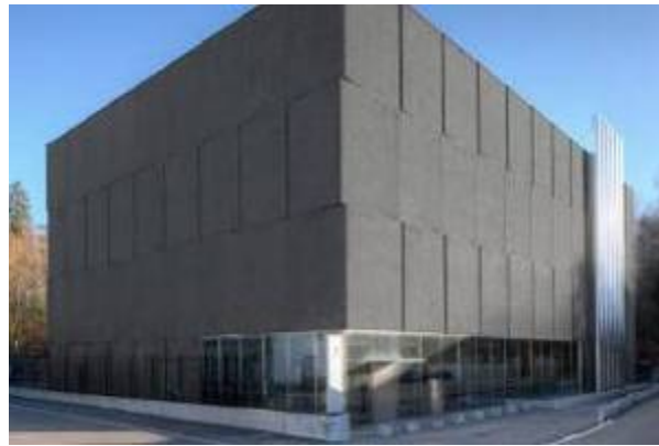
Figure 8: New DC of Swisscom located in the canton of Berne (Switzerland)
